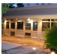
Guard houses & security entrances.
